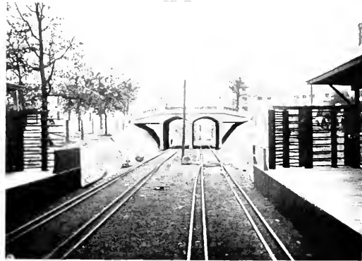
FIG. 3.—STATION ON ELECTRIC RAILWAY.
